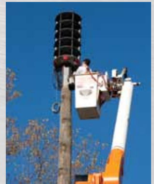
Installation of VisuAlert™ on siren
