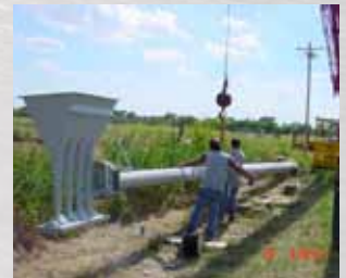
Ohio Valley Installation
