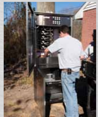
Electronic cabinet installation
