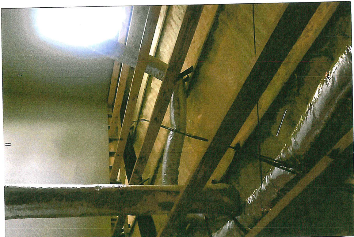
Framing ceiling joists in office areas
