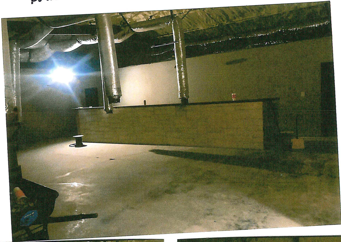
Council room before ceiling project
