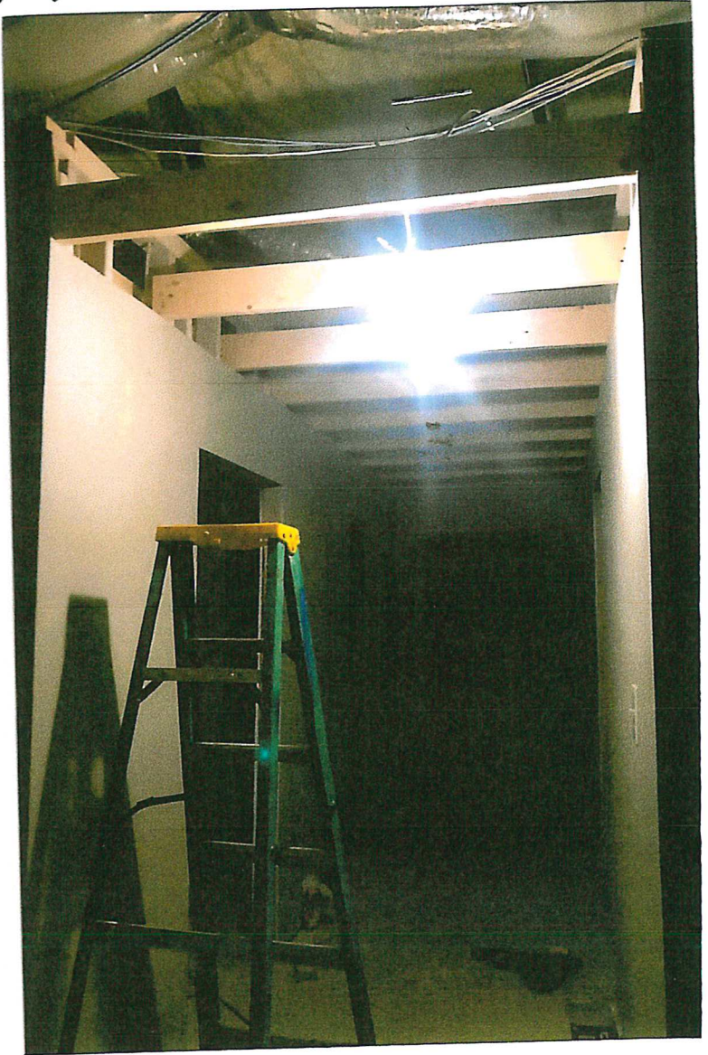
Framing hallway ceiling joists
