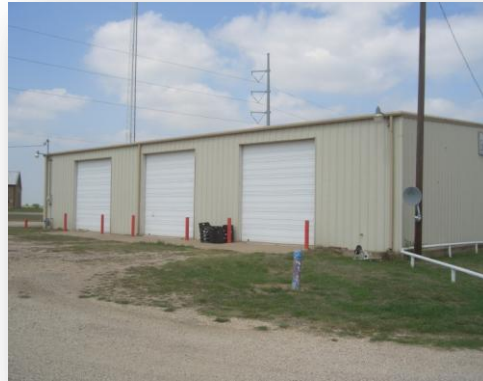
Figure 8-13 Fire Engine Bay
