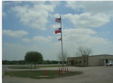
Figure 8-10 Bruceville-Eddy Municipal Building
