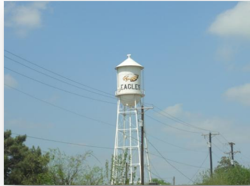
Figure 8-15 Historic Water Tower
