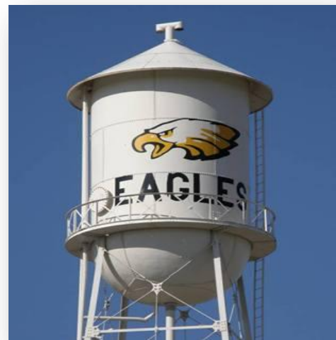
Figure 6-2 Bruceville-Eddy's Historic Water Tower
